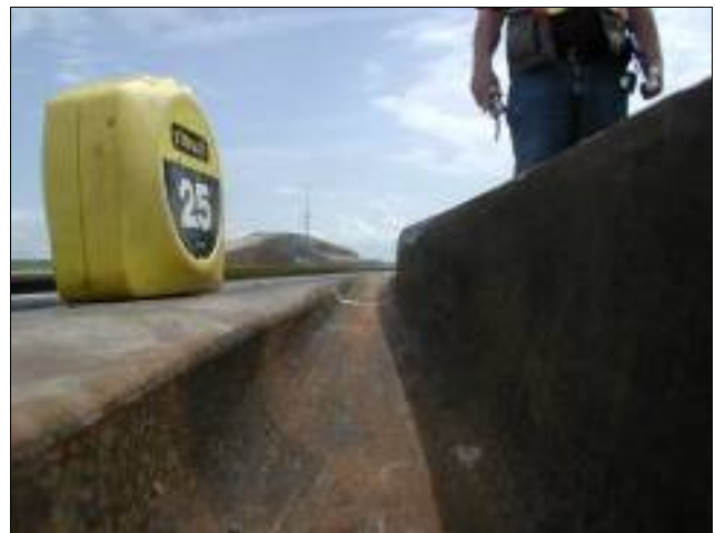
Figure 3. Heel-End Casting of Flange Bearing Turnout Frog
