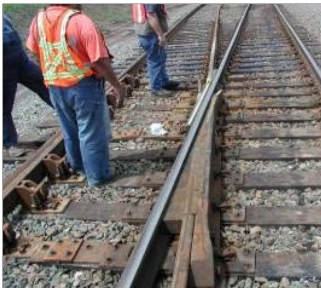
Figure 1. Flange Bearing Turnout Frog (Toe-End View)
