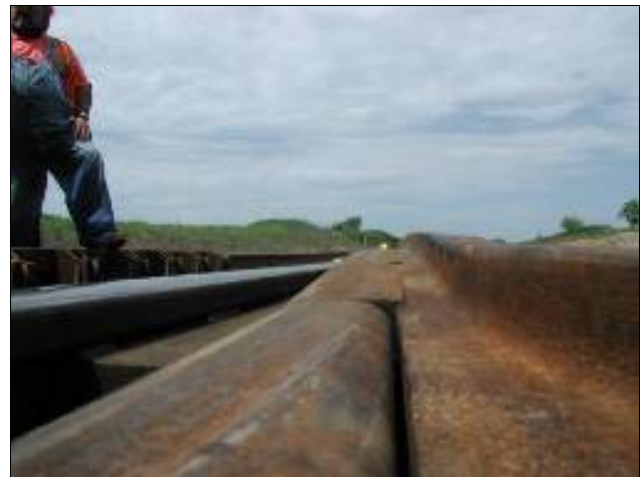
Figure 2. Tread Bearing Ramp on Toe-End Casting
