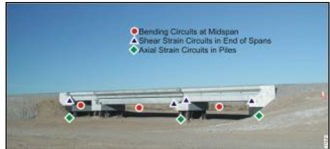
Figure 1a. SOA Concrete Bridge at FAST
