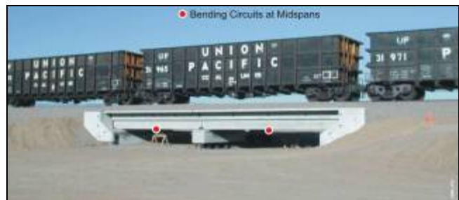
Figure 1b. Conventional Concrete Bridge at FAST
