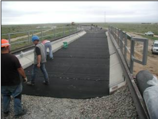
Figure 2b. Ballast Mat during Installation on the SOA Bridge at FAST
