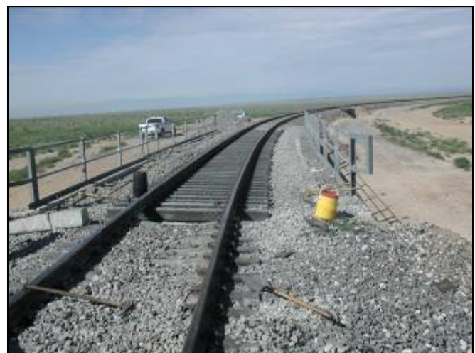
Figure 2a. Plastic Ties on the SOA Bridge at FAST
