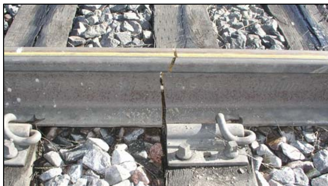
Figure 4. Broken Rail at FAST
