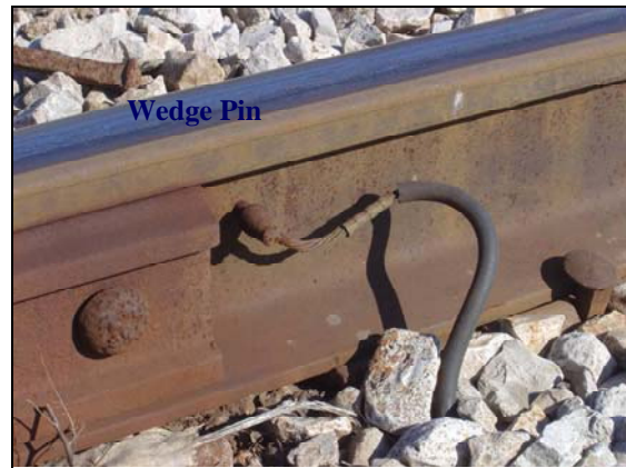
Figure 3. Plug Bond or Chicken Head Track Wire Bond
