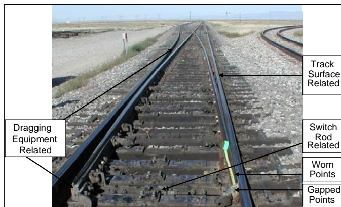
Figure 1. Typical Mainline Switch and Potential Failure Locations
