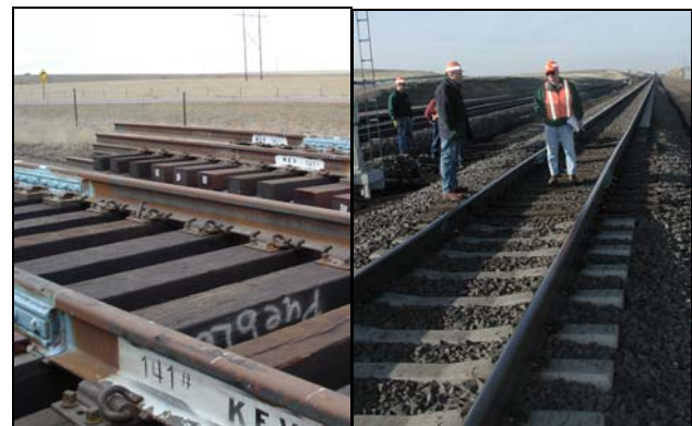
Figure 1. Installation of IJs on Track Panels
