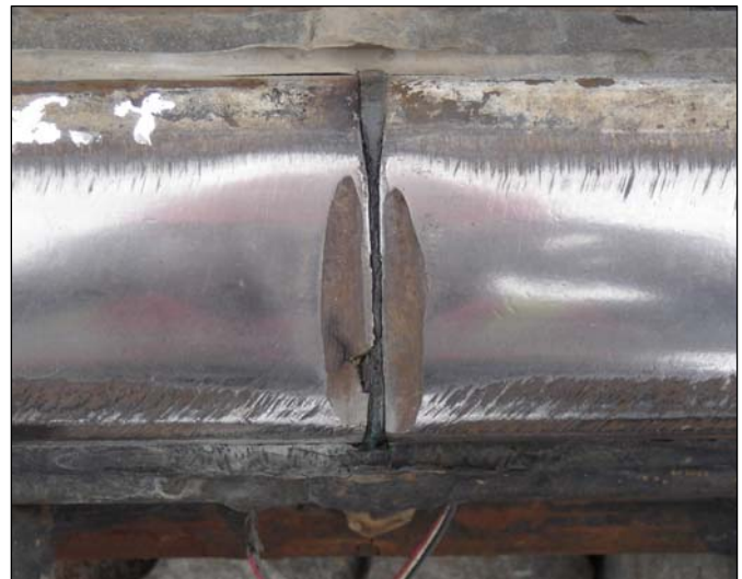
Figure 3. Less than Optimal Joint Slotting
