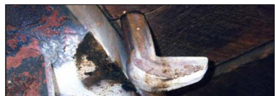
Figure 4. Turned Hook Bolt
