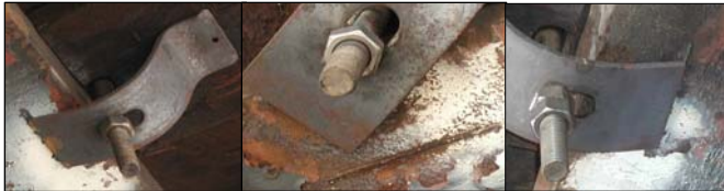
Figure 8a (left). HCP-25 Spring Clip with Single Nut. Figure 8b (center). Rotated Spring Clip and Gouge in Girder Flange. Figure 8c (right). HCP-25 Spring Clip with Double Nuts
