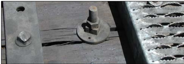
Figure 5. Double Nut and Washer Nut with Nail Hole
