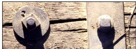
Figure 3. Original Conrail System using a Hook Bolt and a Washer Nut
