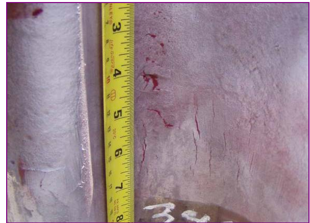
Figure 11. Tears and Gouge on Pulling Face
