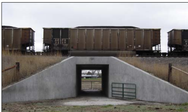
Figure 1. Bridge Approach Test Site
