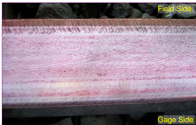
Figure 7a. Post-Grind Rail Surface Conditions, TOR Zone (Low Rail — Curve G, Site 5L)
