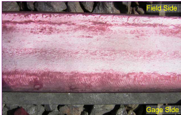
Figure 6a. Pre-Grinding, TOR and Optimized Gage Face Lubrication (Low Rail — Curve G, Site 5L)
