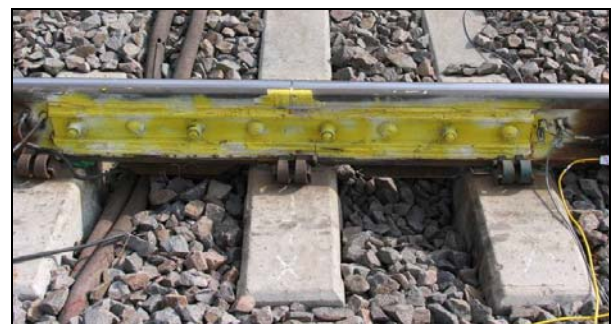
Figure 3. Three-Tie Plate, Direct Support Foundation
