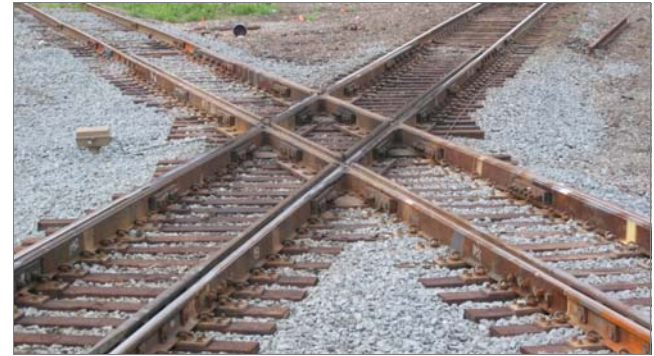
Figure 1. CSX Shelby, OH FBF Crossing Diamond
