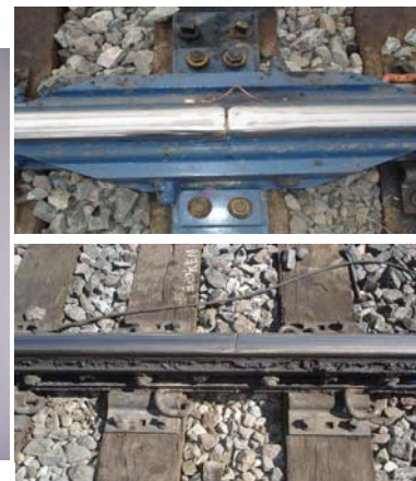
Figure 4 (top) High Modulus Joint Bars 2*RE and (bottom) 1.25*RE
