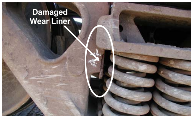
Figure 4. Damaged Truck Side Frame Column Guide Wear Liner
