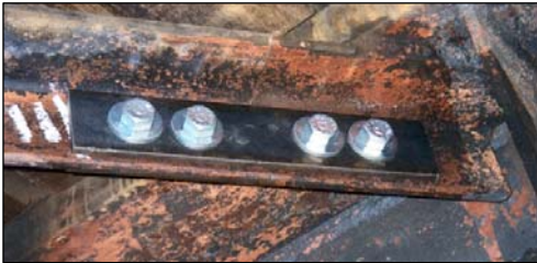
Figure 2. A Lateral Brace in the 65-Foot Span after Repair
