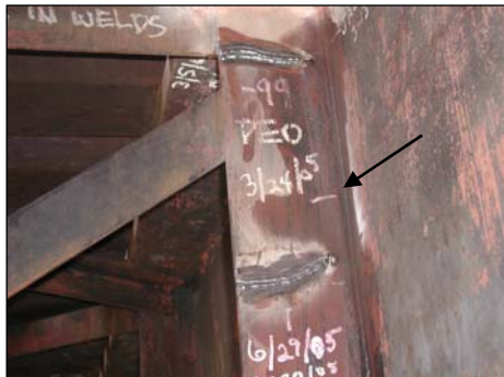
Figure 3. A Stiffener Repaired with Drilled Holes and Additional Weld
