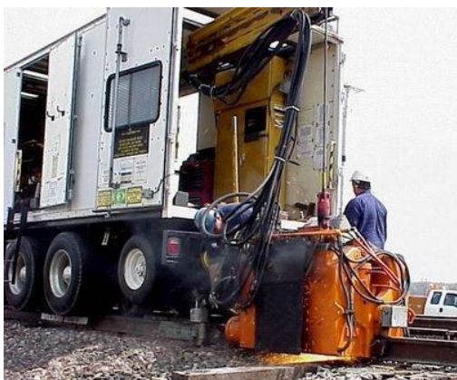
Figure 4. Holland Installing Reduced Consumption Test Welds in Track at FAST
