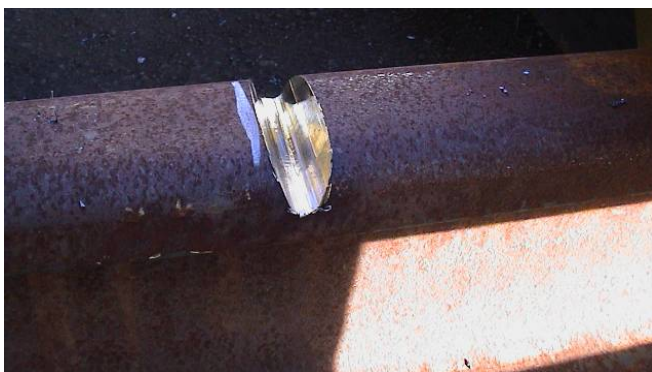
Figure 2. Rail Head Milled for GMAW Robotic Slot Weld
