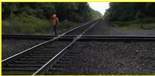
Figure 1. Track Transition at a Diamond Crossing
