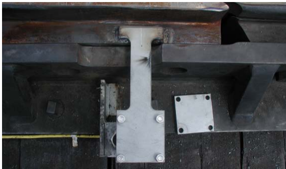
Figure 2: Steel Target and Proximity Sensor, Welded to Miter Joint
