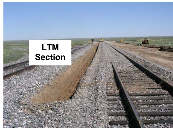
Figure 6. Drainage Trench along the LTM Section
