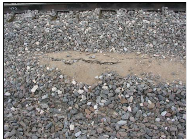
Figure 2. Early Indication of Asphalt Damage
