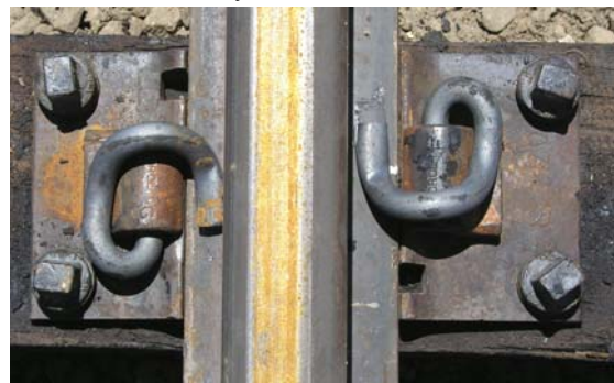
Figure 1a. Top View of the Pandrol Victor ® Elastic Fastening System and LB&N High Strength Screw Spikes
