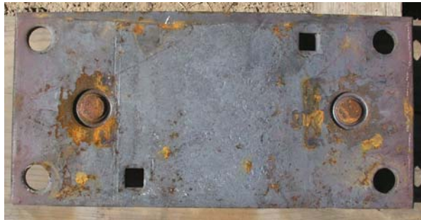
Figures 1b. Bottom View of the Pandrol Victor® Elastic Fastening System
