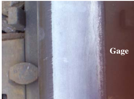
Figure 8. Low Rail Contact Region Shifted from Rail Shoulder to Crown Region
