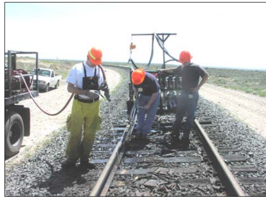
Figure 1. Willamette Valley Company's Push-Type, Single-Gun Machine in a Wet Installation Sub-zone
