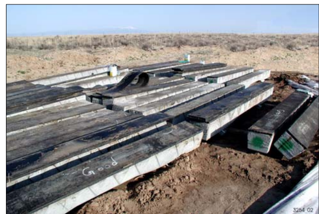
Figure 2. Concrete Ties with Rubber Pads prior to Installation at FAST
