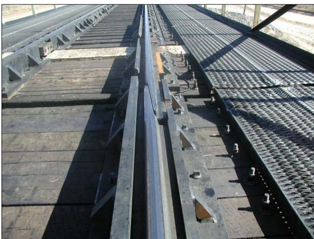
Figure 1: Amtrak Long-Point Thick-Web Bridge with Joints Installed
