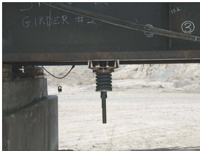
Figure 3: Hold Down for Lifting Rails
