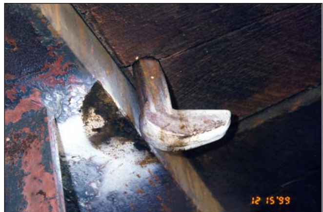
Figure 2: Turned Hook Bolt
