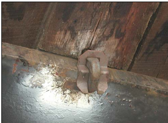
Figure 4: Hook Bolt with Locking Clip
