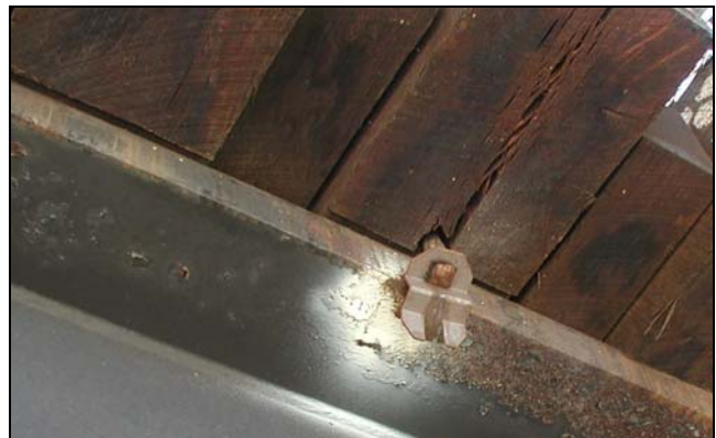
Figure 6: Broken Hook Bolt with Locking Clip
