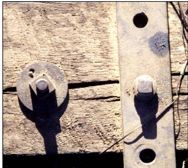
Figure 1: Original Conrail System using a Hook Bolt and a Washer Nut with a Nail through the Washer Nut to Prevent Rotation
