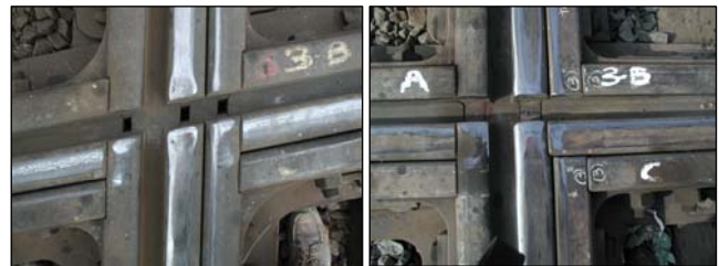
Figure 2. Conventional and Herringbone Rail Arrangements at Diamond Frog
