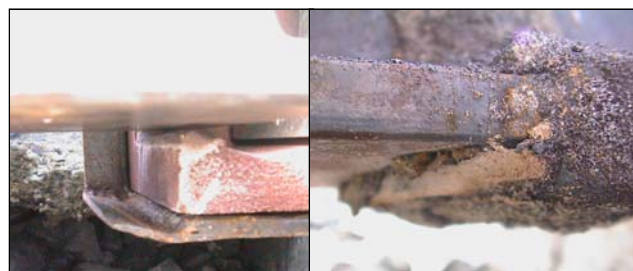
Figure 5a: Rail bottom and weld mold with refractory paste 1
