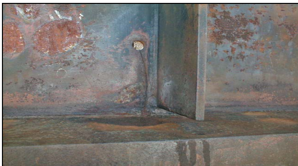
Figure 4. Crack in the Flange
