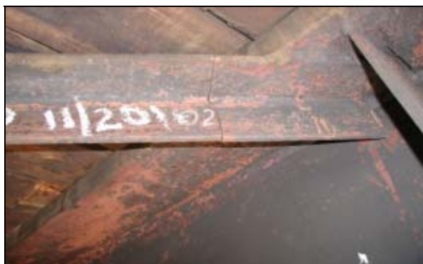
Figure 4. Crack in the Flange
