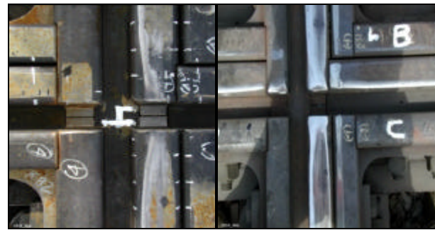
Corner 4 Ramp at 5 MGT Corner 4 ramp at 81 MGT Figure 4: Ramping System –Diamond Crossing Minimal Deformation after 81 MGT at the Ontario Site
