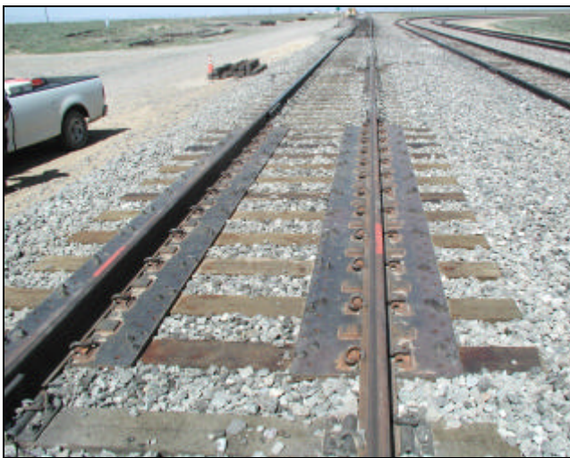
Figure 4. Damping Test Panel Installed at FAST
