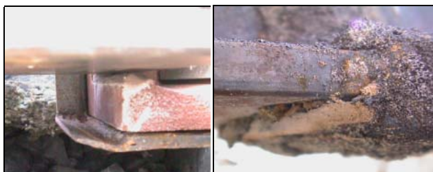
Figure 4a: Rail bottom and weld mold with refractory paste.
