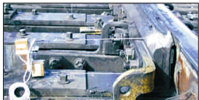
Figure 6. Measuring Switch Point Roll under Traffic
