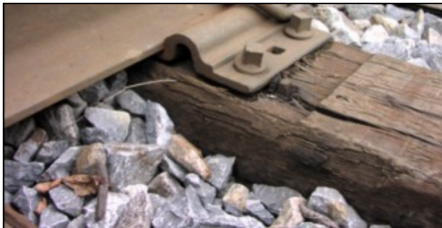
Figure 2. Elastic Fastening System Installed on Old Ties
