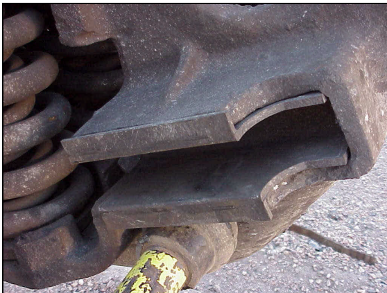
Figure 2. Brake Beam Pocket with Plastic Wear Liner showing Smooth Wear Surfaces with No Gouges or Ridges — Car 97405
