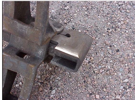
Figure 3. Brake Beam End Extensions Showing Typical Normal Wear Patterns — Car 97405
