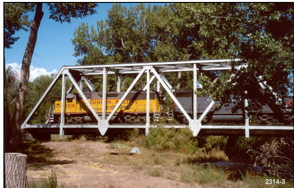
Figure 6. Single-Span Through Truss Test Bridge on UP at Cañon City, Colorado
