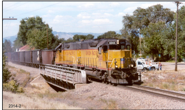
Figure 5. Single-Span TPG Test Bridge on UP at Florence, Colorado
