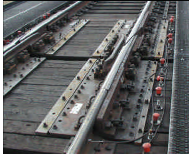
Exhibit 1. AMS Casting Bridge Joints Installed
