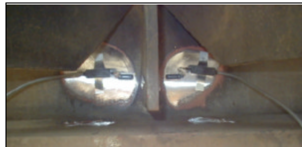
Exhibit 1. Strain Gages Attached to Backside of Girder Web
