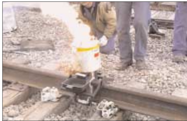
Exhibit 3. Test Weld being Poured at FAST for Laboratory Evaluation
