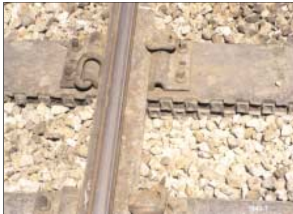
Exhibit 2. USPL Plastic Ties with Roughened Surfaces and Elastic Fasteners in HTL Section 7
