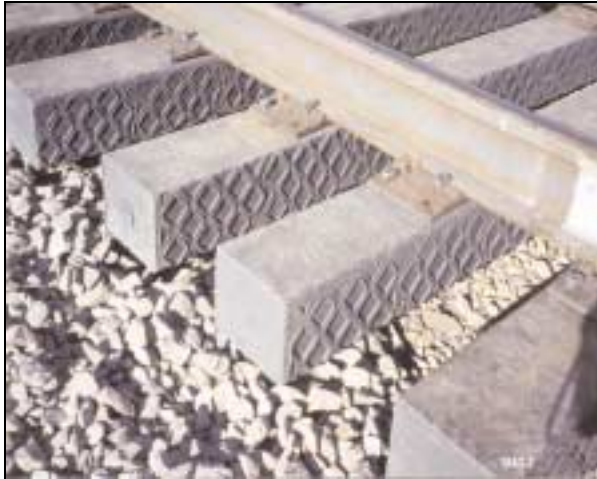
Exhibit 1. TieTek™ Plastic Ties with Roughened Surfaces, Fastened with Cut Spikes in HTL Section 25
