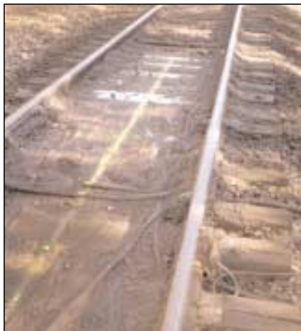
Exhibit 2. Yellow Paint Mark on Tangent Track at a Wayside Lubricator Location
