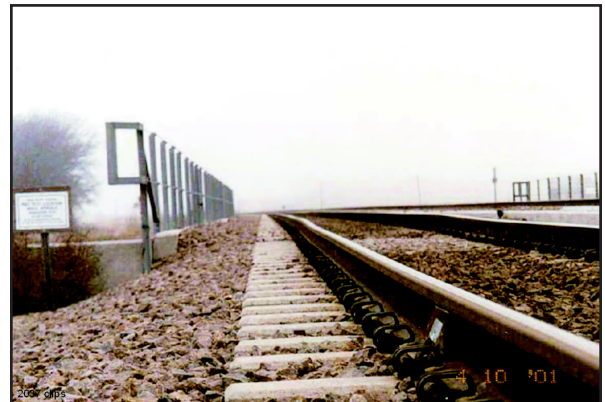
Exhibit 3. Track Surface on HMA Approach Bridge Prior to Surfacing
