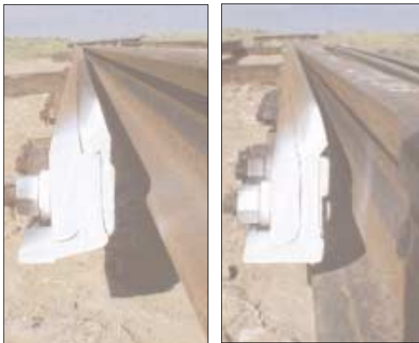
Exhibit 1. TTCI Prototype Switch Profile vs. AREMA Switch Profile
