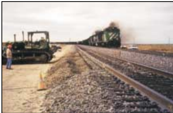
Exhibit 2. Track Buckle Test in Progress
