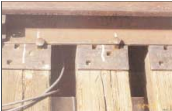
Exhibit 3. Intermediate Span – Deck and Girder Movement
