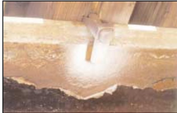
Exhibit 8. End Span – Hook Bolt to Top Flange
