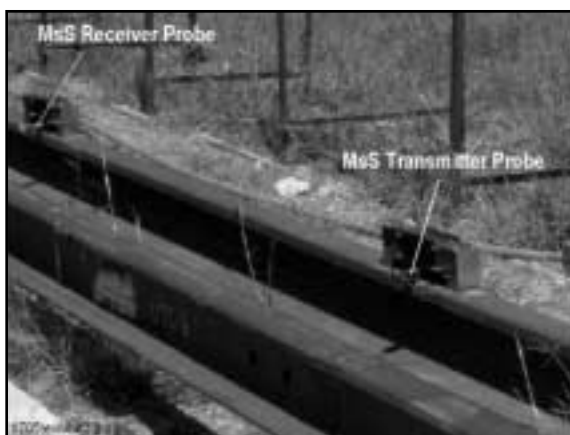
Exhibit 2. Placement of MsS Probes on Sample Rail to Determine Guided Wave Behavior (MsS Probes are Sitting on Railhead and Covered with Permanent Magnets)
