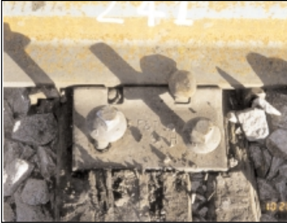
Exhibit 3. Tie-Plate Cutting and Loose Screw Spikes in Phase V
