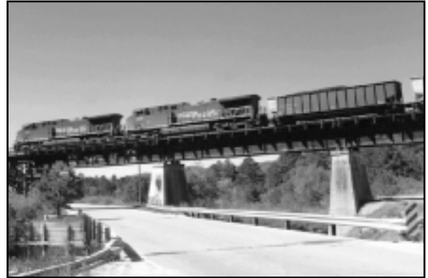
Exhibit 1. UP Coal Train Crossing BNSF Test Bridge
