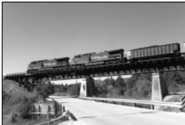
Exhibit 3. AC Locomotives Crossing Bridge
