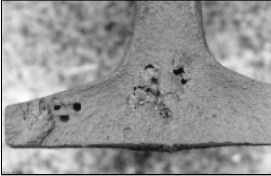
Exhibit 5. Thermite Weld with Slag/Porosity
