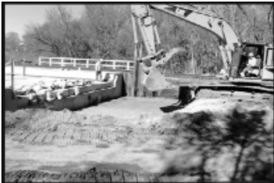
Exhibit 3. Installation of Concrete Stabilized Soil Approach
